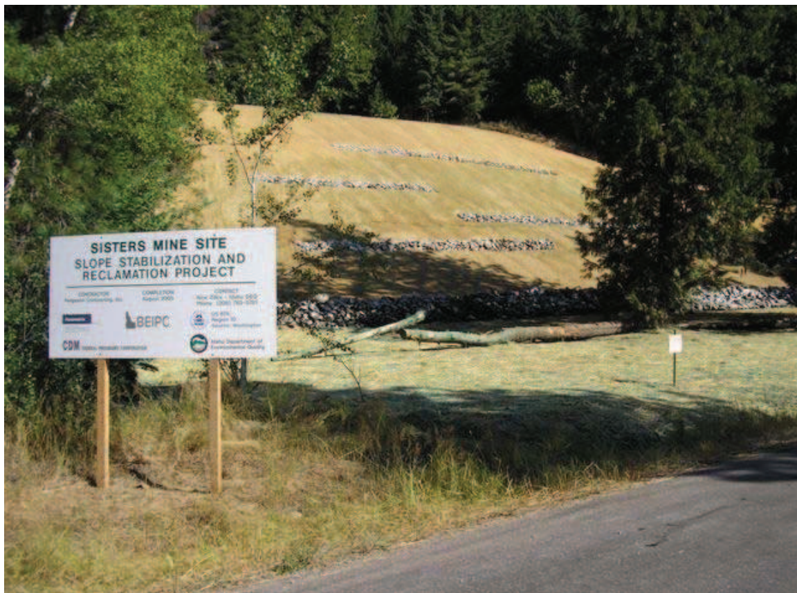
Sisters Slope Stabilization at completion of project
