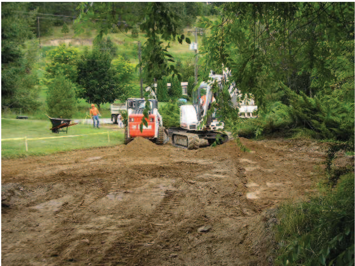
Coeur d'Alene Basin Property Remediation
